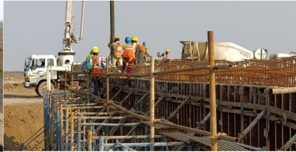
E-3 BRIDGE: SUBSTRUCTURE CONCRETING
