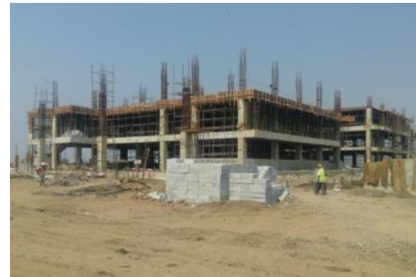
BEC 2 nd Slab Shuttering
