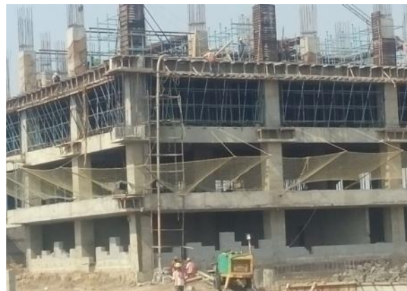
SPV Building 4 th floor column progress
