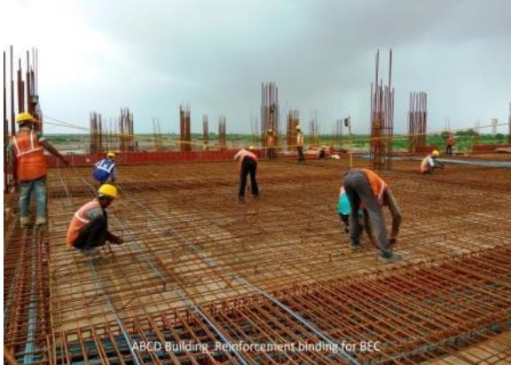
Reinforcement for BEC Slab
